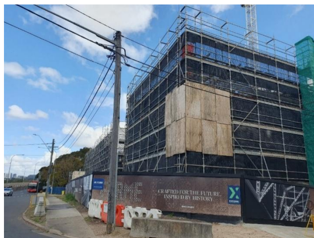
Figure 3 - Subject site as viewed from the corner of Church Street and Well Street
