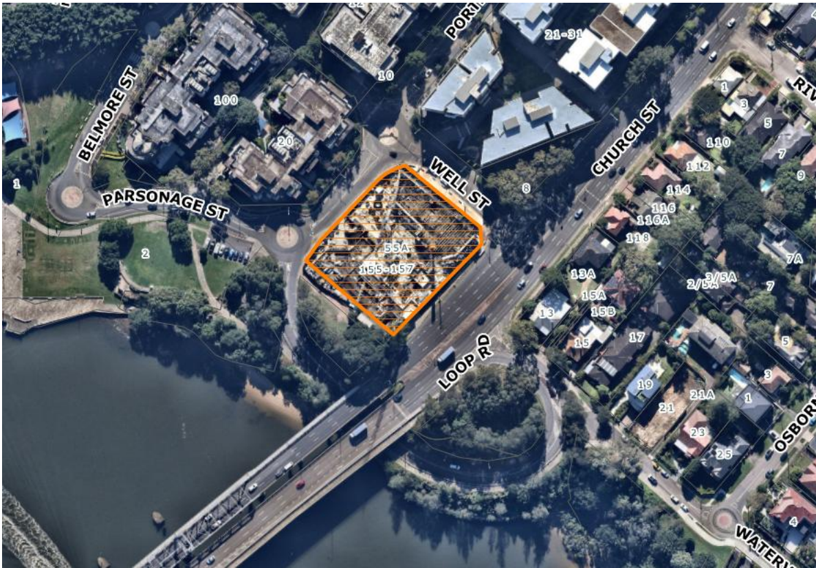
Figure 2 - Aerial photo of the site and surrounds. The development is currently under construction.
